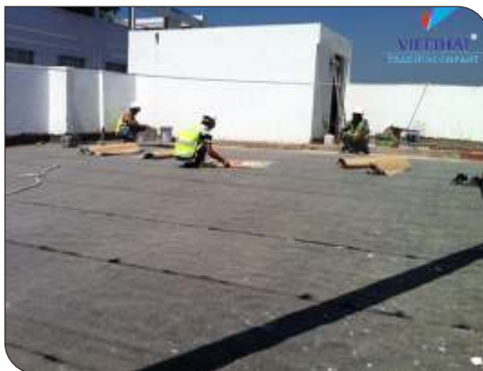
Applying self-adhesive membrane
