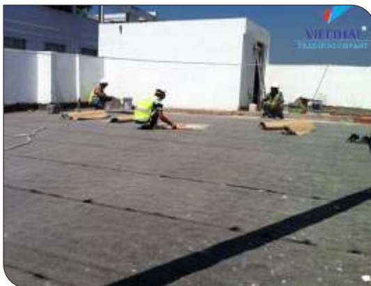
Applying self-adhesive membrane
