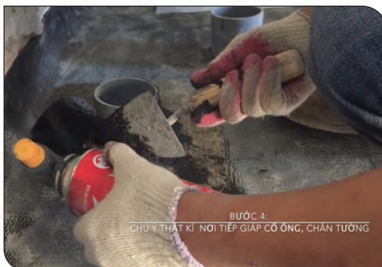
Treating the neck of the drain pipe
