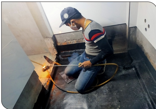
Construction of torched on membrane
