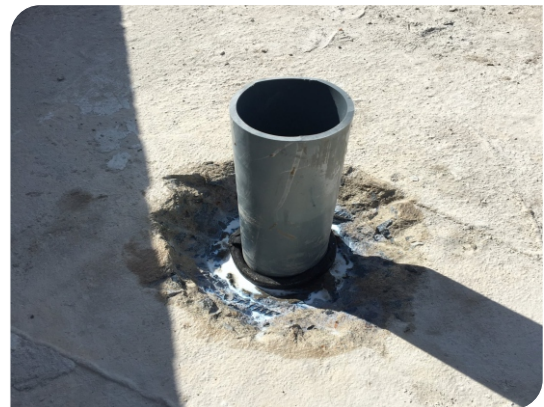
Clean the neck of the pipe, wrap the expansion tape
