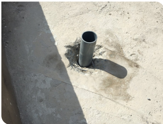
Beveled around the neck of the pipe
