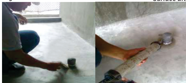
Apply BS 8620s glue to seal the gap around the downpipe
