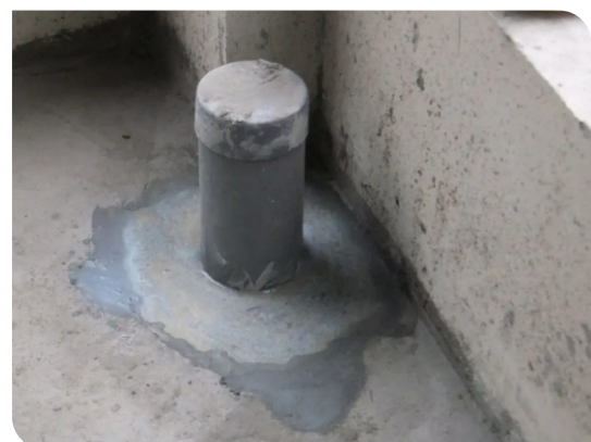
Surface after grouting
