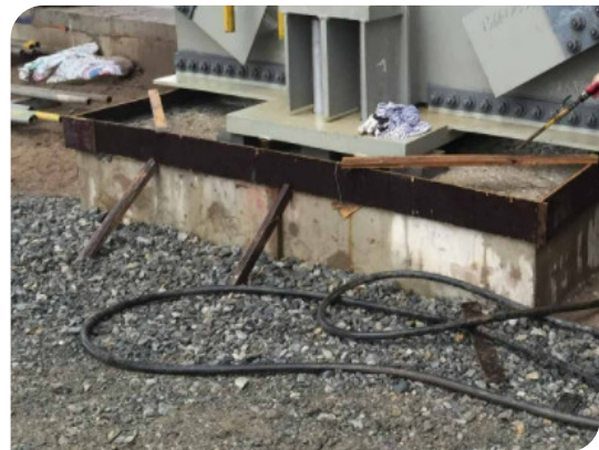
Installation of formwork
