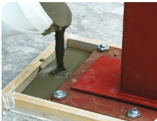
Grouting construction
