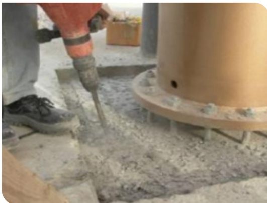
Chisel to roughen the surface
