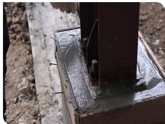
Column base after grouting
